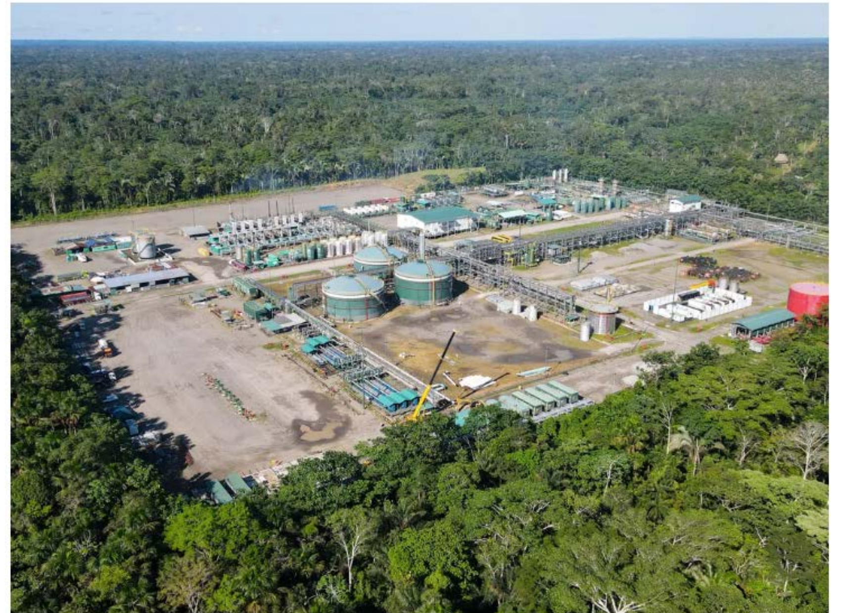
Aerial view of the Tiputini Processing Center of state-owned Petroecuador in Ecuador's Yasuni National Park photo courtesy of Rodrigo Buendia/AFP via Getty Images.
